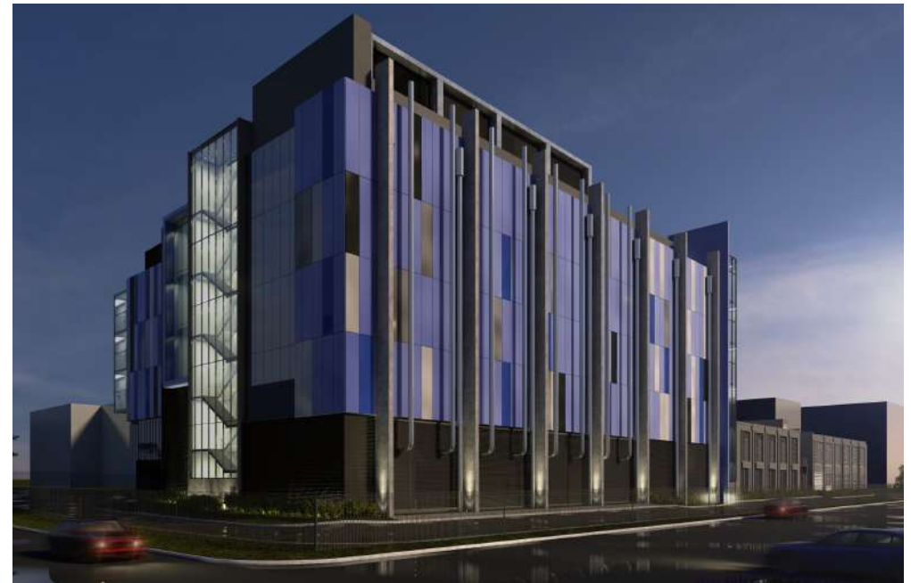
Macquarie Data Centres is adopting a more flexible approach in preparation of future expansions of their data center.
